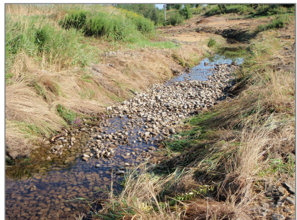
One of six projects included restoration of 1,700 linear feet of Penjajawoc's stream channel. Photo: City of Bangor
