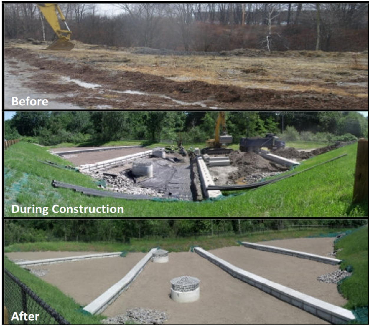
Installation of soil media filter during Mall Plaza Phase. I
